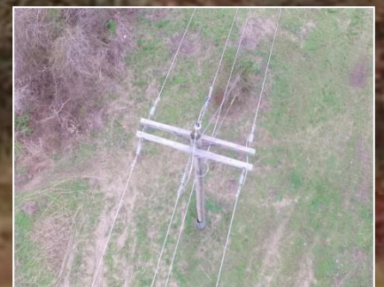
POLE TOP INSPECTION
